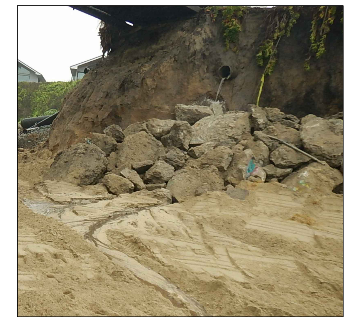
PICTURE 3 WEST SIDE OF BRIDGE IN THE CREEK FACING EAST
