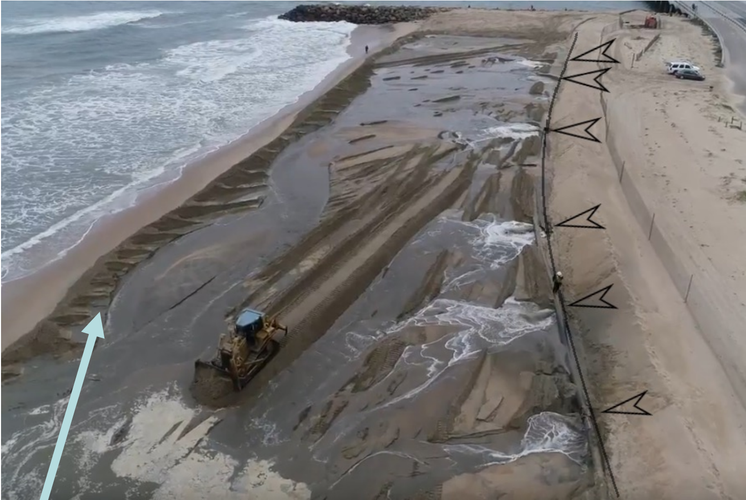
Sand Containment Berm
