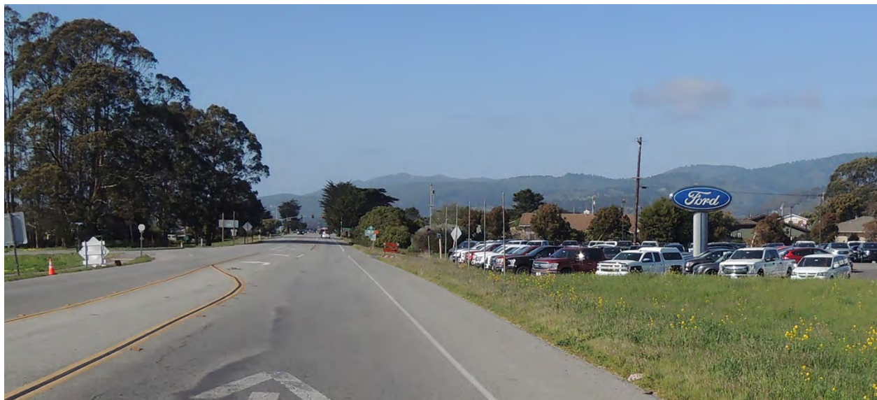
Figure 1-5 Existing Conditions at Location 2
