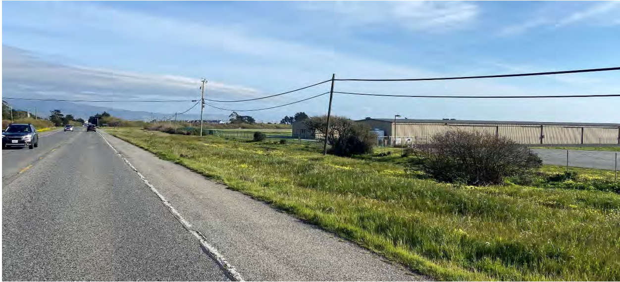
Figure 1-13 Existing Conditions at Location 5
