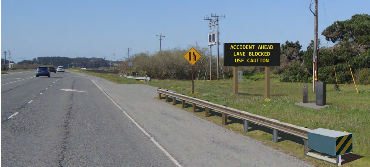
Figure 1-19 Visual Simulation of VMS (shown with message displayed), MVP and MGS at Location 6
