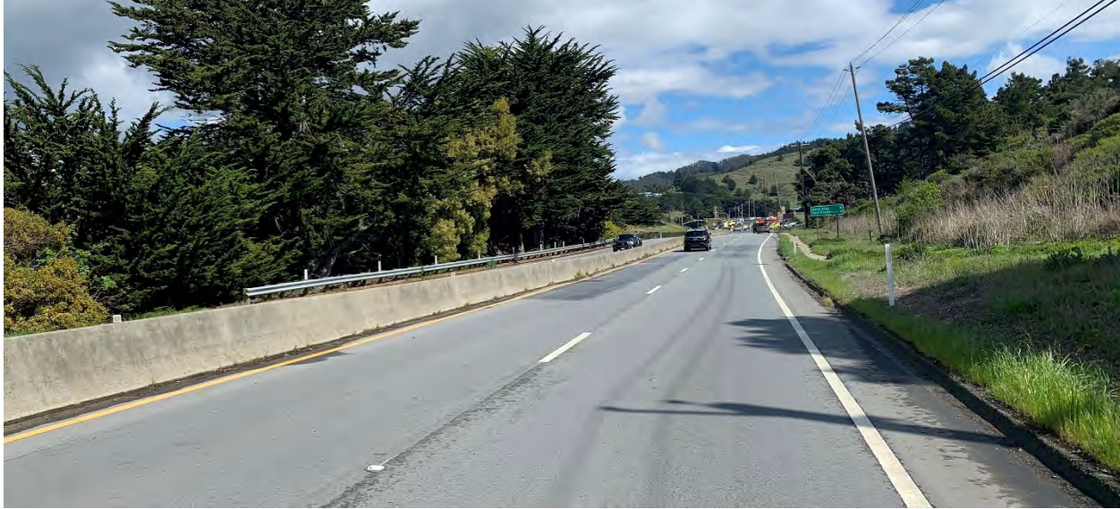
Figure 1-26 Location 9-2 Existing Conditions
