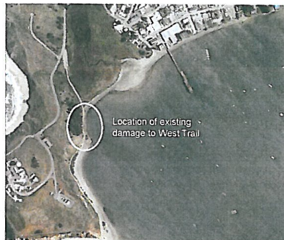
Figure 1. Location of West Trail damage
